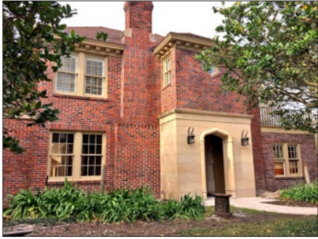
The exterior of 913 Sorrento Road before the renovation
