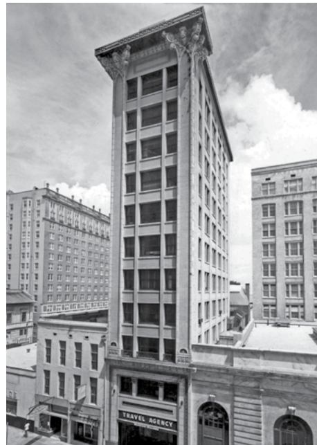
The Florida Life Building before its beautiful Sullivanesque capitals were destroyed in 1994. Photo provided by Judy Davis.
