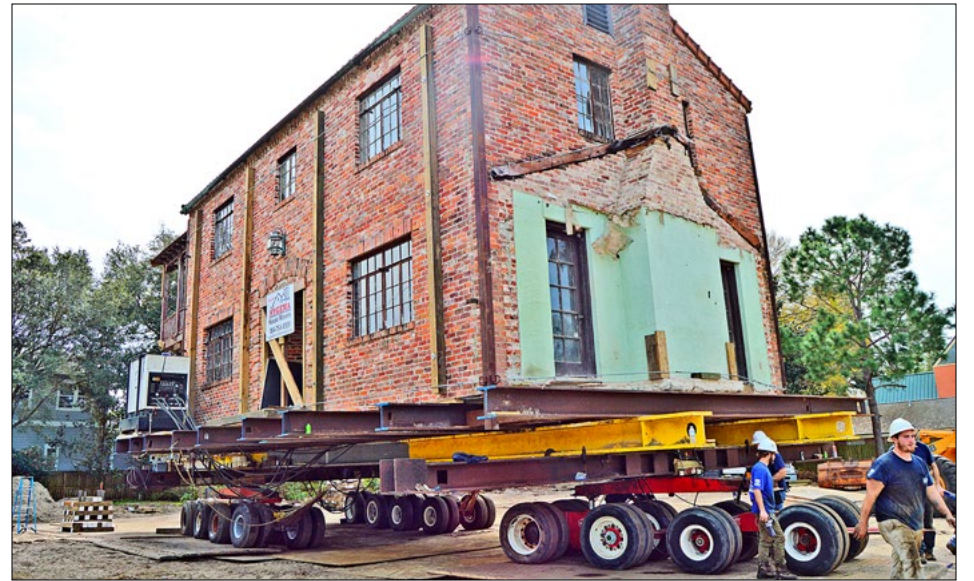
The historic home that formerly resided at 4001 San Jose Blvd., at the corner of Eutaw Place and San Jose Boulevard, has been turned 90 degrees and moved 150 feet so it will face Eutaw Street.
