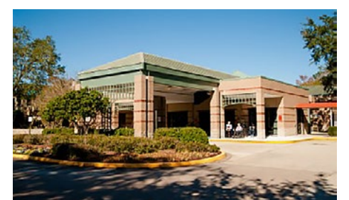
River Garden Hebrew Home celebrated 30 years at its current location. This is how the location looks today.
