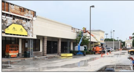
Crews make visible progress on transformation of Ortega Park.
