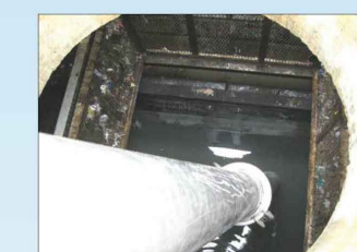
Open lower screen panels to remove sediments via vacuum.
