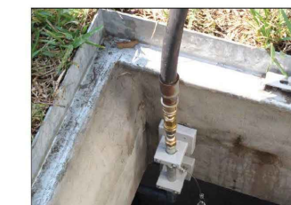
HydroSlide™ quick connector with vacuum truck water supply hose attached for sediment removal.
