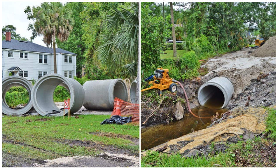
Underground piping will bury the creek from Olga Place to Sydney Street
