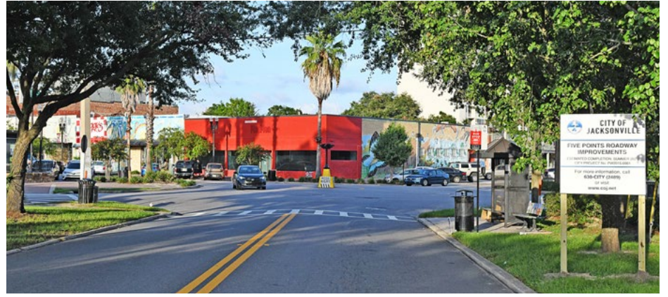
The approach to 5 Points, seen here from Park Street, will change as construction begins Aug. 31 on the streetscapes during the execution of the 5 Points Concept Plan.
