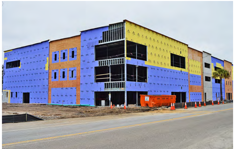
Progress is being made on the building of a new storage facility on the old Jones College campus in Murray Hill.
