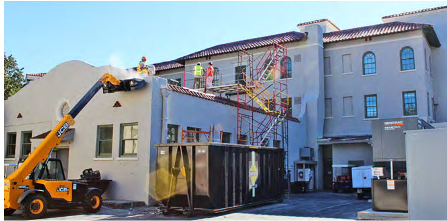
Thanks to a generous gift from the Gund family, renovations are being made to transform the second floor of Bolles Hall into a girls' dormitory
