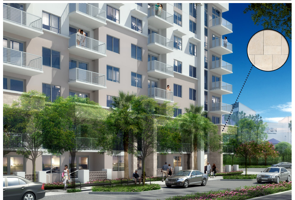
TOP RIGHT IMAGE: Updated renderings of the East facing façade, the direction facing St. Johns River Park and the Friendship Fountain was a large question mark for DDRB board members. Related Group team members went back to the drawing board and provided relief [or façade projections, versus flat fronted] along this portion of the development along with other measures - to the pleasure of the voting board – and subsequent approval.
