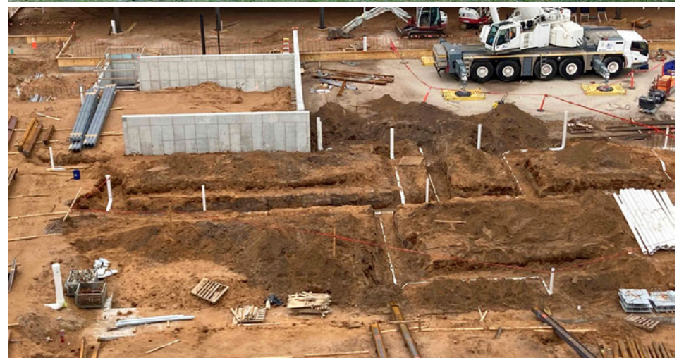
Construction is moving along at a clip at the site of the new JEA Headquarters. The new, 135,000-square-foot-building will have a Pearl Street address.
