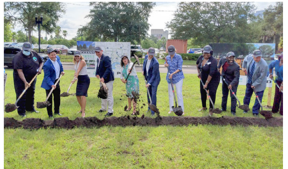
Stakeholders engaged in the Emerald Trail project tossed dirt to celebrate the first phase of the trail getting underway.
