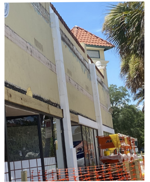
1950 San Marco Blvd. gets a fresh coat of paint
