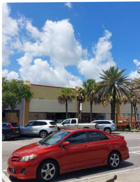
1950 San Marco Blvd. during renovations
