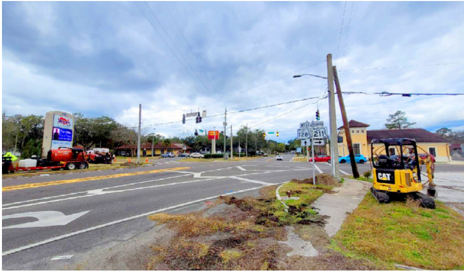
Duval Asphalt Products begins work on San Juan Avenue.
