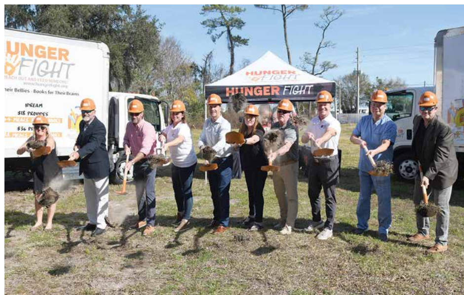
On Jan. 20, 2023, Hunger Fight's top supporters were captured tossing the dirt at the site of the new headquarters on the corner of St. Johns Bluff and Airport Terrace Drive.
