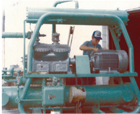
James "Dan" Griffin, Jr. August 1979 working on a G500 Chiller
