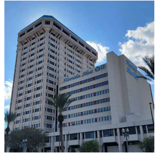
New office space for JSO Homeland Security Division will soon be available at the Florida Blue Building on Riverside Avenue.
