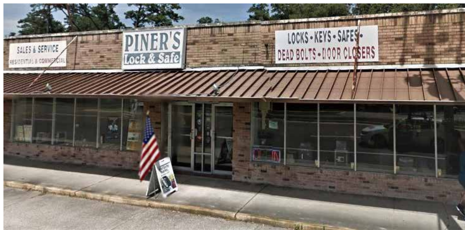
Piner's Lock & Safe anchored the old Miramar Plaza shopping center for years before Vega closed the storefront in March 2020.
