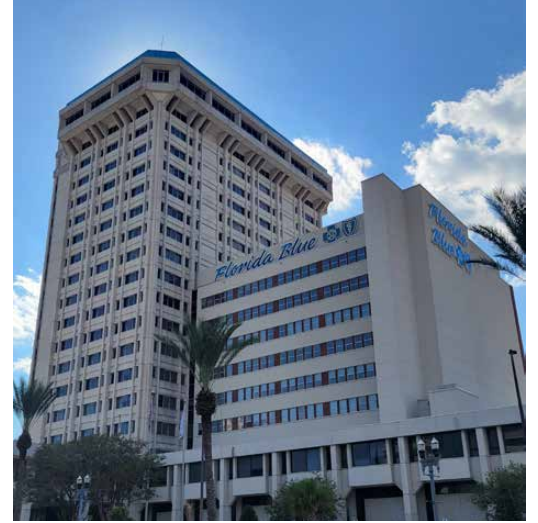
New office space for JSO Homeland Security Division will soon be available at the Florida Blue Building on Riverside Avenue.
