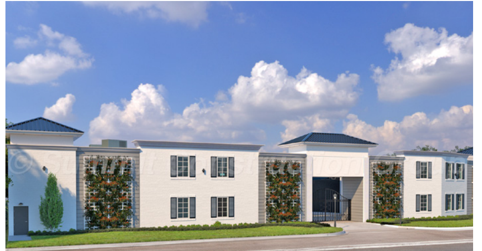
The proposed Ortega Carriage House project would run along Ortega Boulevard with its main entrance off Manitou Avenue.
