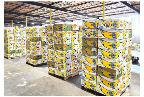
The new facility provides both warehouse and refrigeration space as well as room for more than 100 volunteers at a time to receive, sort and package more than 34 million pounds of food each year.
