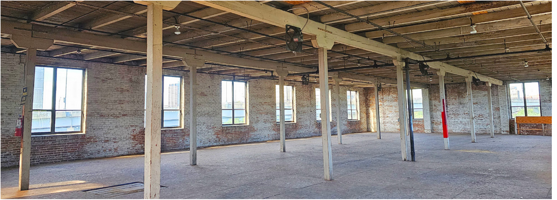
Afternoon sunlight streams through the once bricked-over southwest windows of the Florida Casket Company building as work continues at the Jacksonville History Center.
