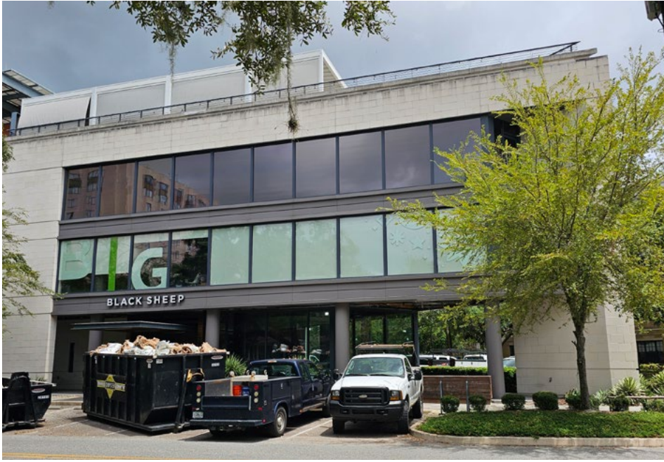
Work is underway at 1534 Oak S. for Bartaco in 5 Points.
